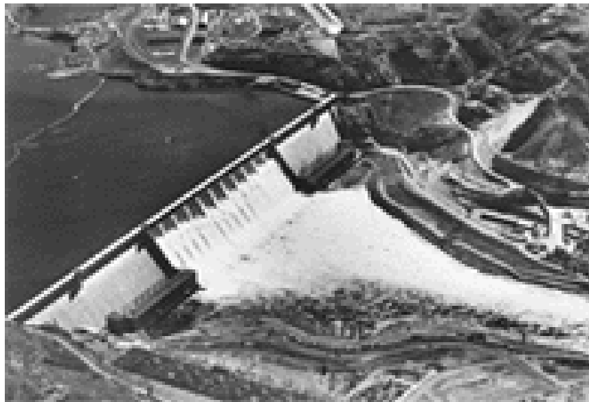
Grand Coulee Dam Columbia River, Washington
